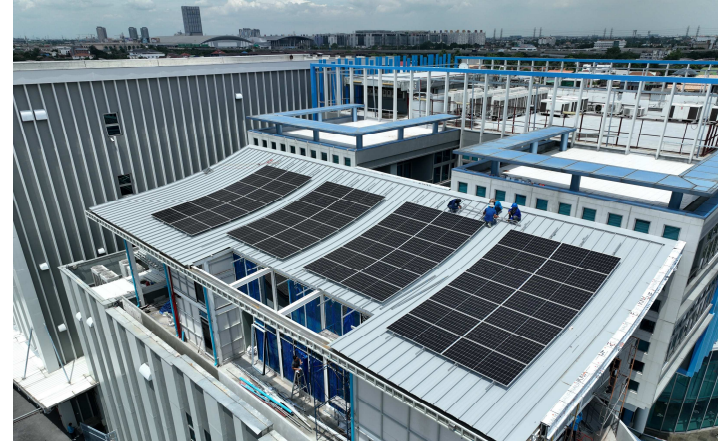
National ITMX (Data Center)
