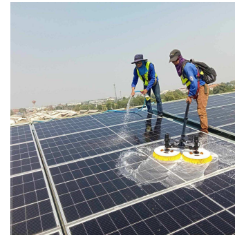
Cleaning PV Module
